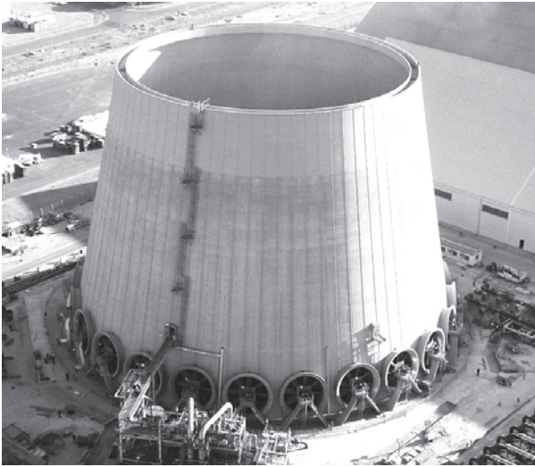
Figure 6 — Fan-assisted natural draft tower.
