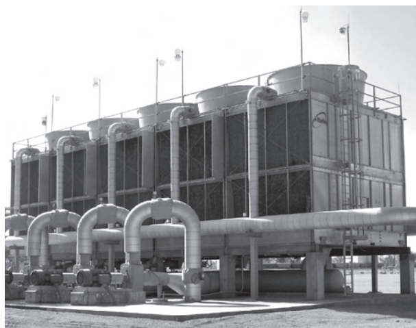
Figure 12 — Multi-cell factory-assembled tower.
