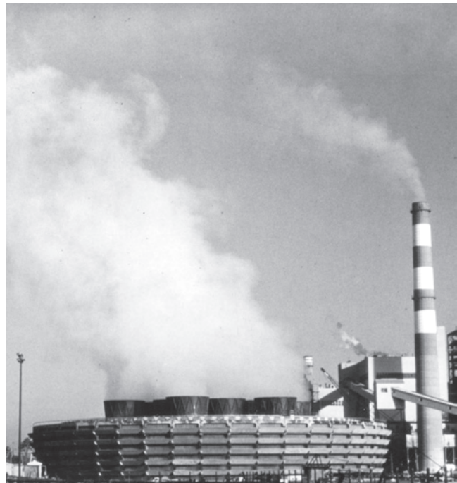
Figure 32 — Round mechanical draft tower operating in a significant wind. Compare plume rise to flat trajectory of smoke leaving stack.
