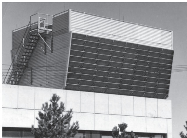
Figure 75 — Casing extended to handrail height.
