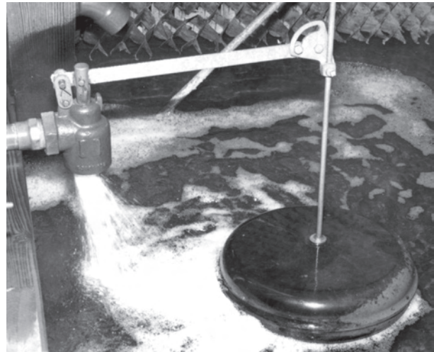
Figure 65 — Float-operated mechanical make-up valve.
