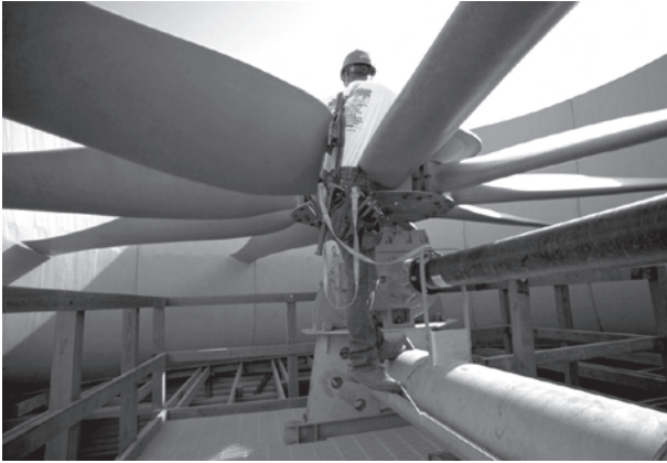
Figure 80 — Large fan being installed.
