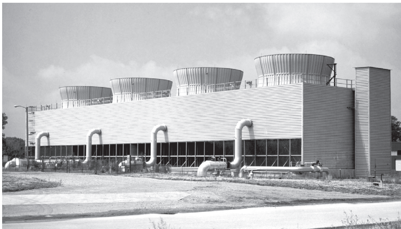
Figure 58 — Four-cell tower with individual side risers.
